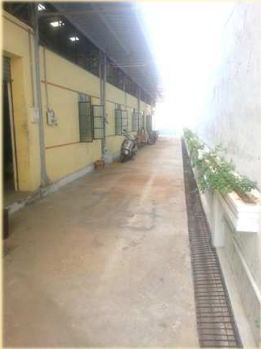
Multi Utility Works Space
